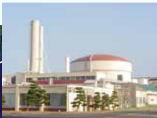
JRR-3@Japan Atomic Energy Agency (20MW Research Reactor)
